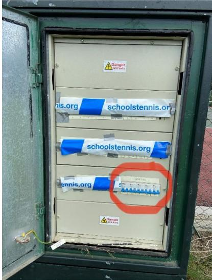
The court number is identified under the switch, push blue switch up to turn on and down to turn off.
